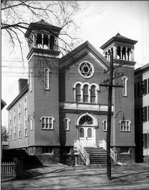
Congregation Ahabat Sholom, original building on Church Street Photo courtesy of Lynn Public Library
